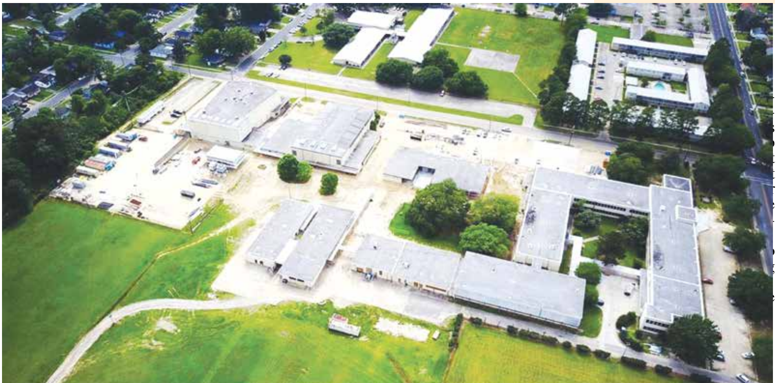
AERIAL VIEW OF ISTROUMA HIGH SCHOOL where construction is almost complete on the newly-renovated school.
