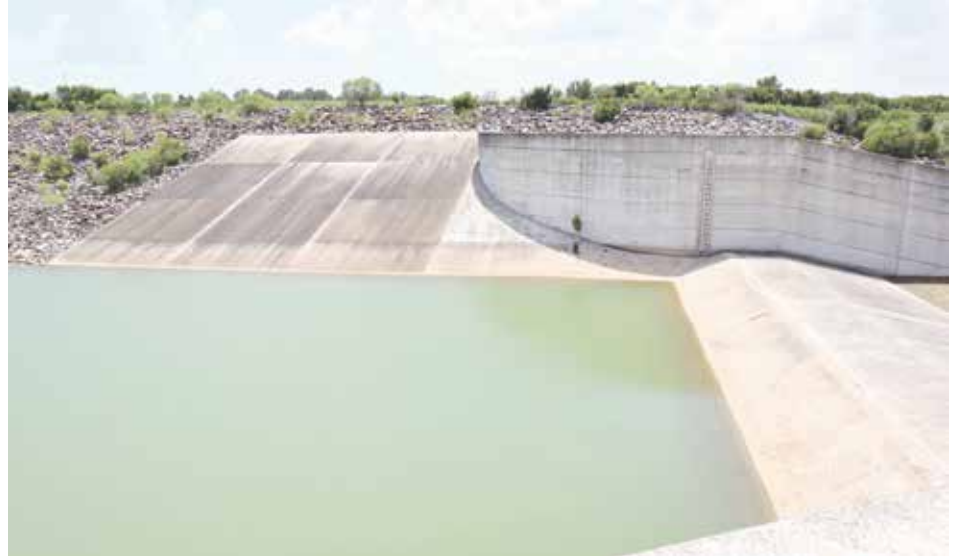
When the Comite tops this weir at 53 feet ASL, flood waters will flow to the Mississippi.
